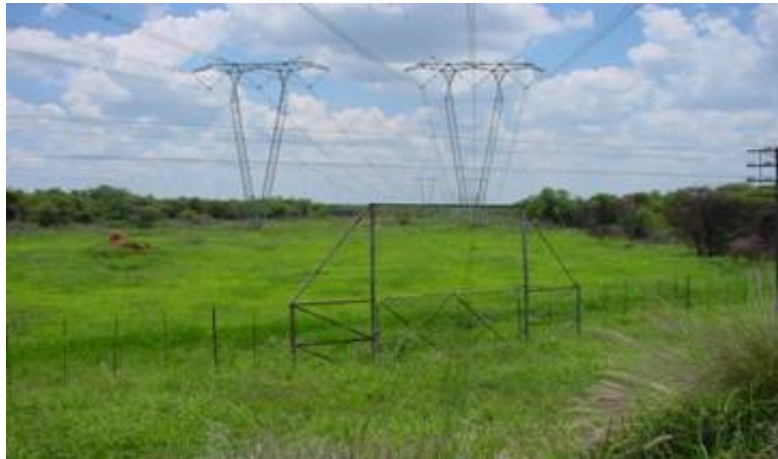
Figure 3.10: Gate Erection (access for maintenance phase) (Step 8)
