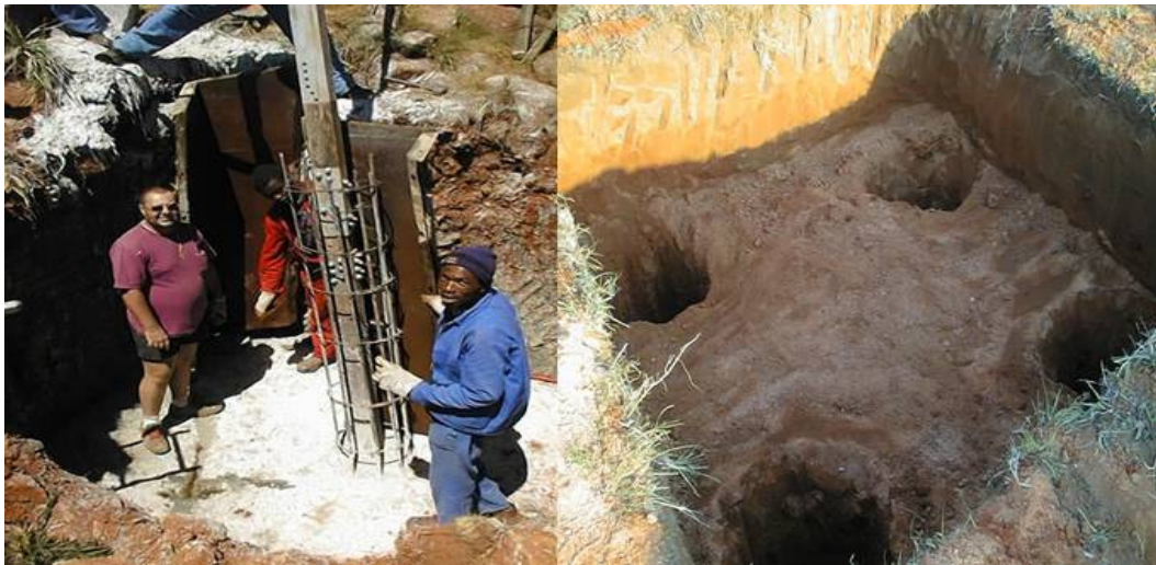
Figure 3.13: Construction of tower foundations (Step 11)
