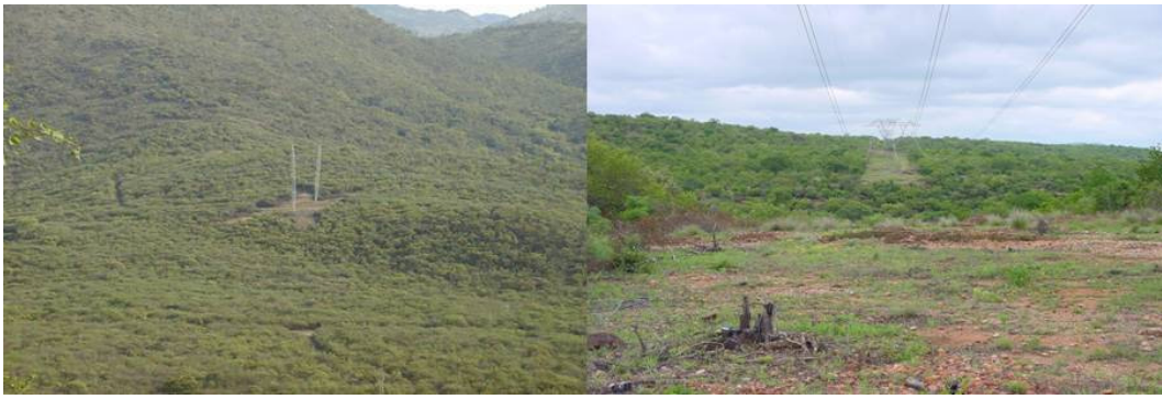
Figure 3.9: Vegetation Clearance (Step 8)
