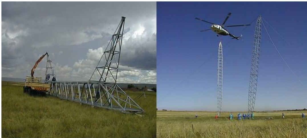
Figure 3.14: Assembly and Erection of towers (Step 12)
