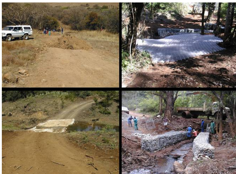
Figure 3.16: Maintenance – Erosion Control
