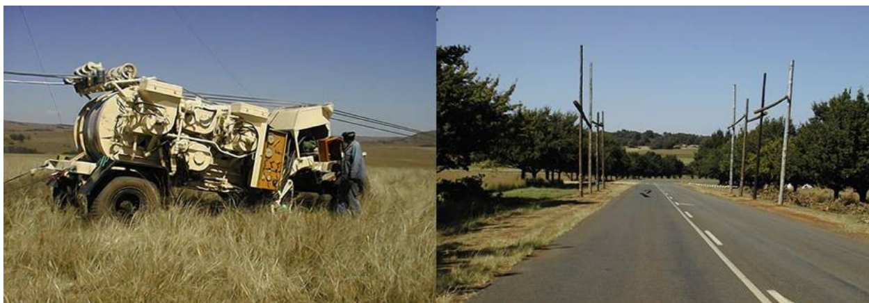
Figure 3.15: Stringing of conductors (power lines) (Step 13)
